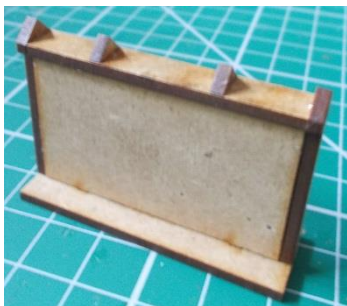
Glue the triangular supports in place.
